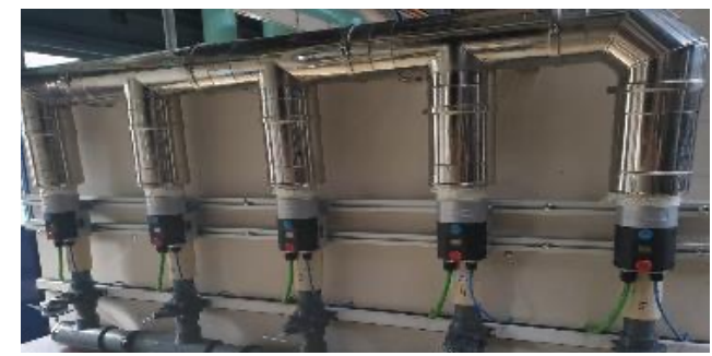
500 kW air heater (up to 600 °C)
