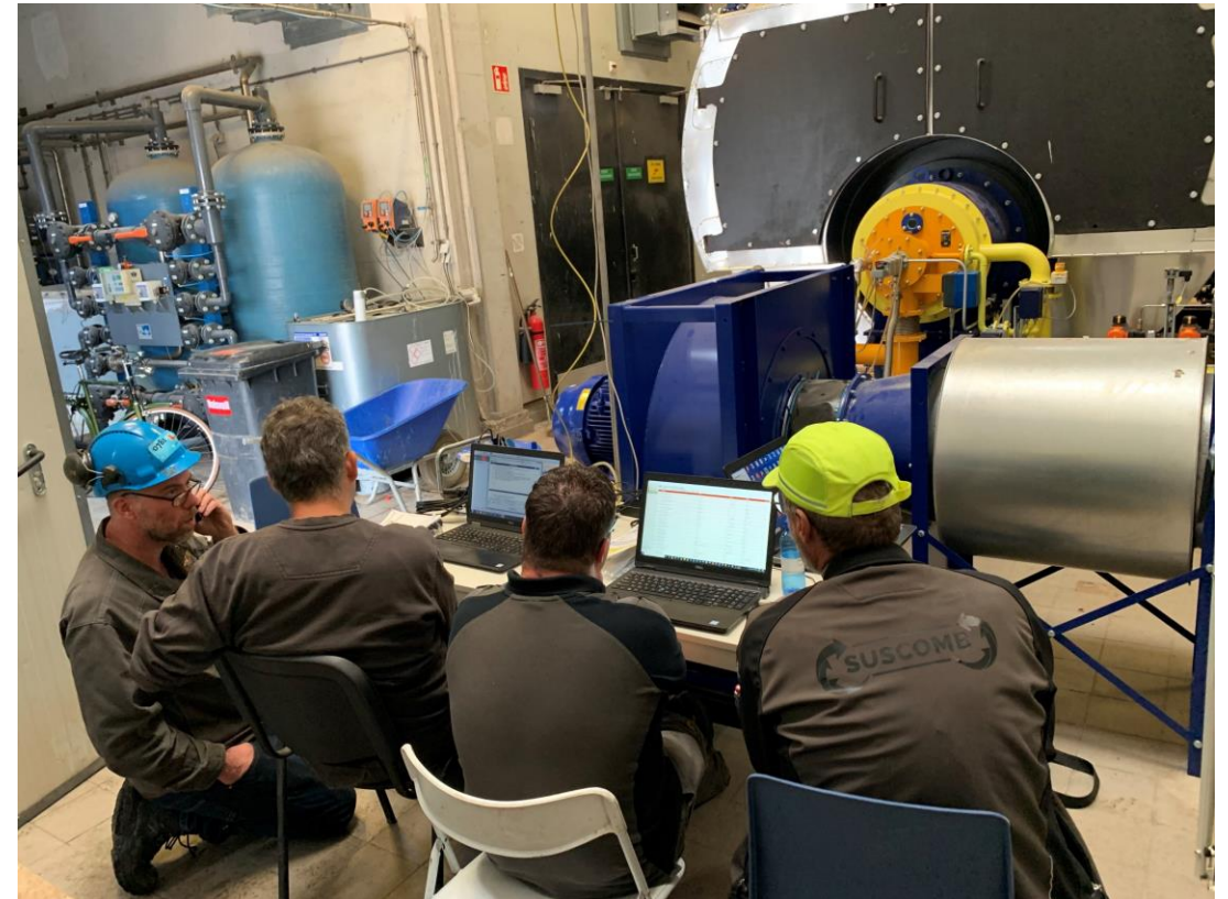
Commissioning SMARTNOX burner by SUSCOMB and Mateq Process
