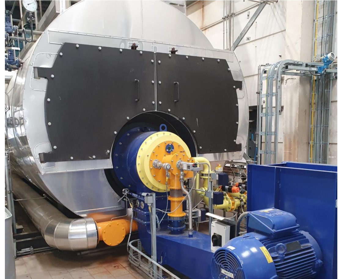
SUSCOMB / Mateq Process 30mg SMARTNOX burner in 7.5MW natural gas firetube boiler
